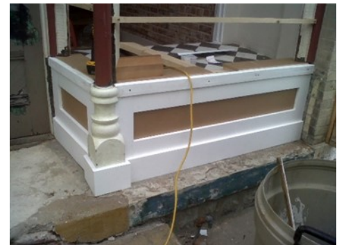
Traditional Hardwood Recessed Bulkhead
