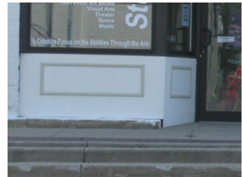
Poor-Quality Substitute Plywood Bulkhead
