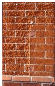
Impact of Blasting/Water/Mismatched Mortar
